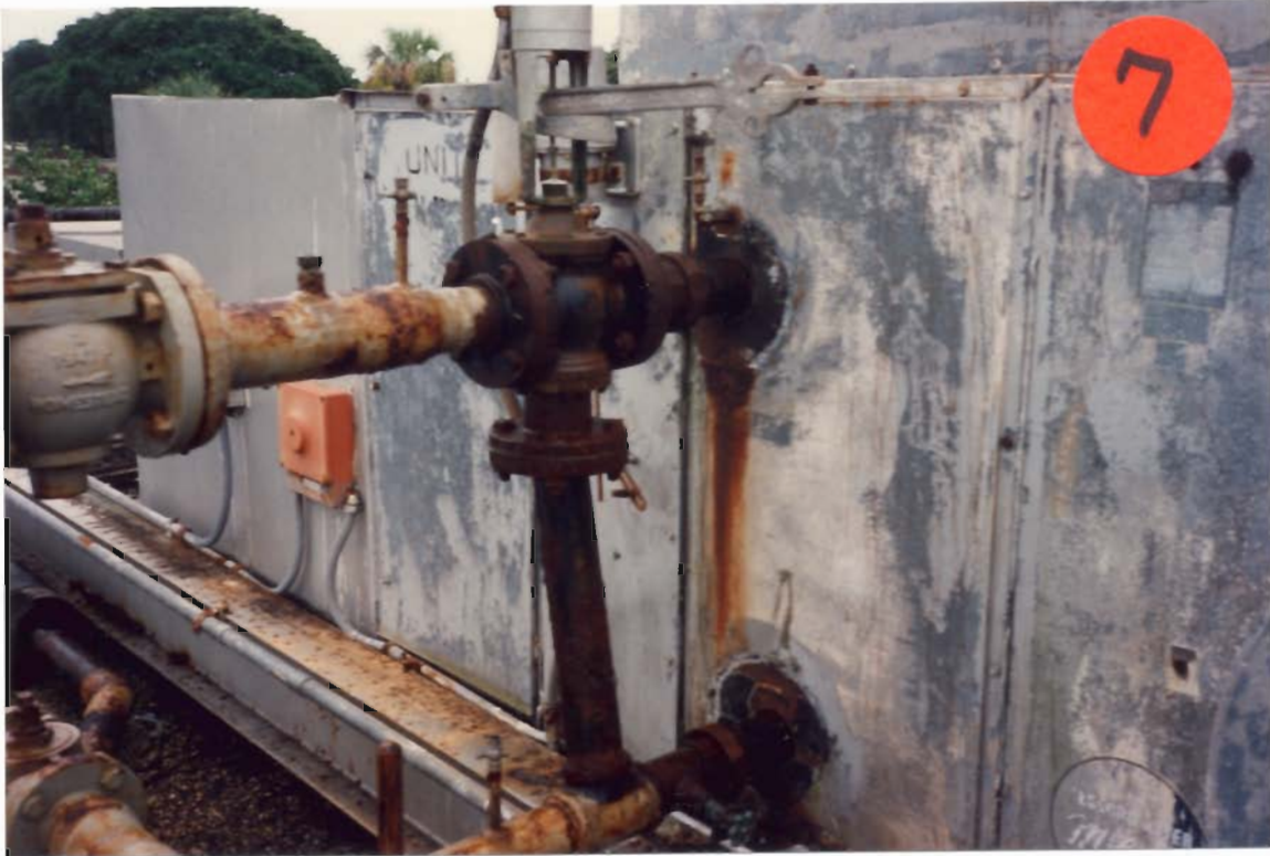
Photograph 8: Clamp On Beam That Has Rusted Into Position Such That The Access Panel To Service This Roof Top Unit Cannot Be Serviced
