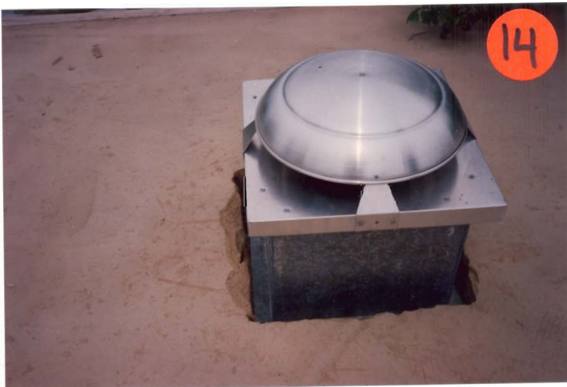
Photographs 14-17: Unprotected Roof Penetrations. Old Rusty Tools And Equipment Were Left On Roof At Job Site
