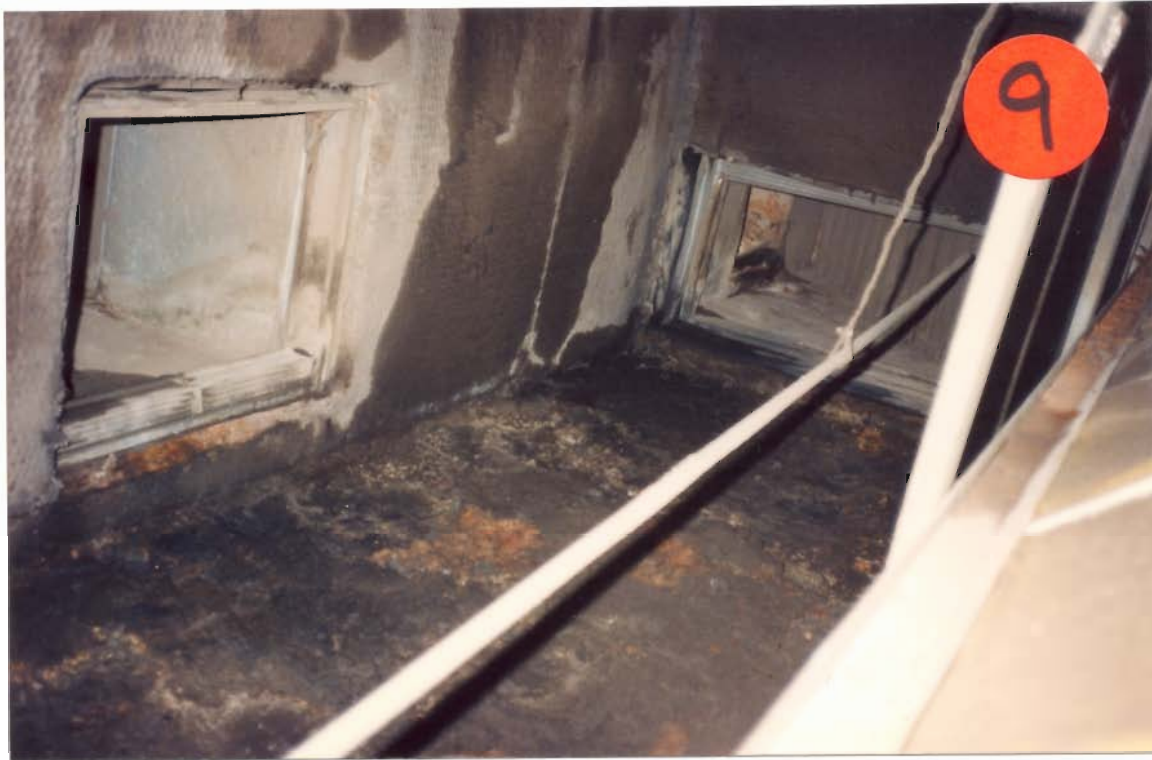
Photograph 10: Rusted Out Top Layer Of Air Handler That Has Collapsed Onto Filter Rack
