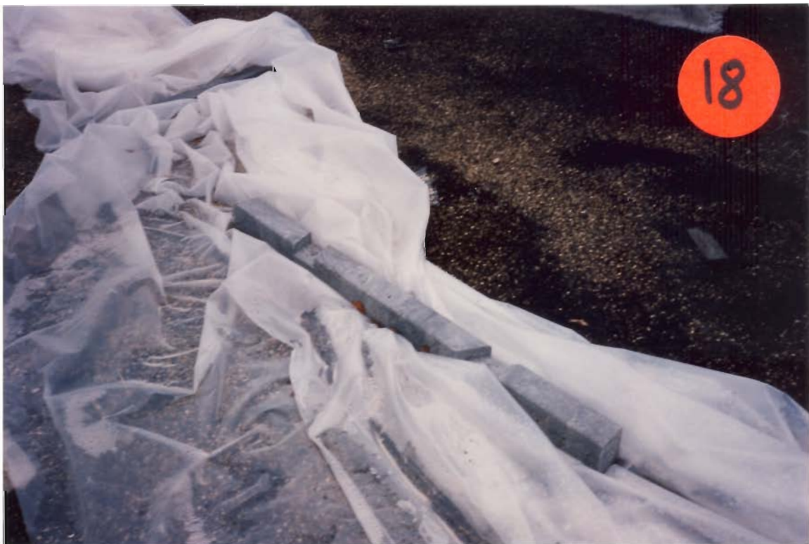
Photographs 18 & 19: Roof Covering And Plastic Sheets On Roof That Were Not Used To Cover Penetrations From Rain
