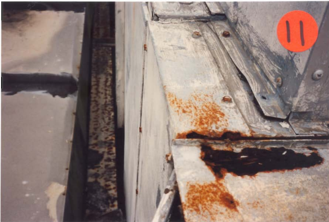
Photograph 12: Very Dirty And Rusty Condensation Pan
