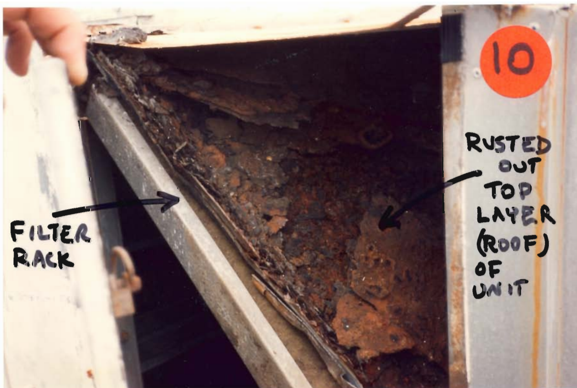
Photograph 10: Rusted Out Top Layer Of Air Handler That Has Collapsed Onto Filter Rack
