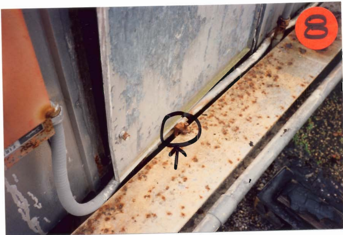
Photograph 8: Clamp On Beam That Has Rusted Into Position Such That The Access Panel To Service This Roof Top Unit Cannot Be Serviced
