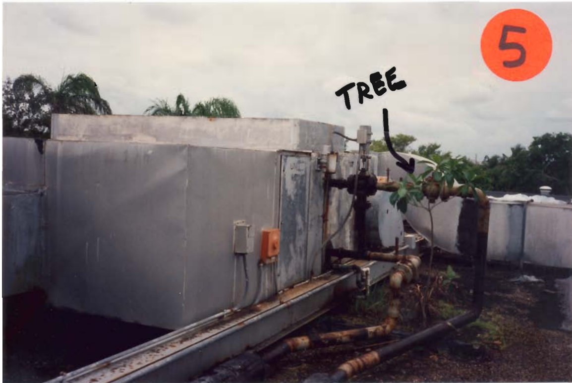
Photograph 6: Large Amount Of Dried Black Mold In Area On Roof Around Outside Air Intake. These Areas Should Be Cleaned Periodically And, If Possible, The Reason For The Inadequate Drainage Corrected
