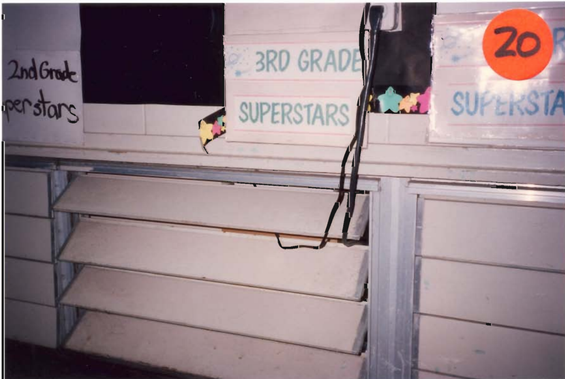
Photograph 20: Unsafe Wiring Practice From One Room To Another Space
