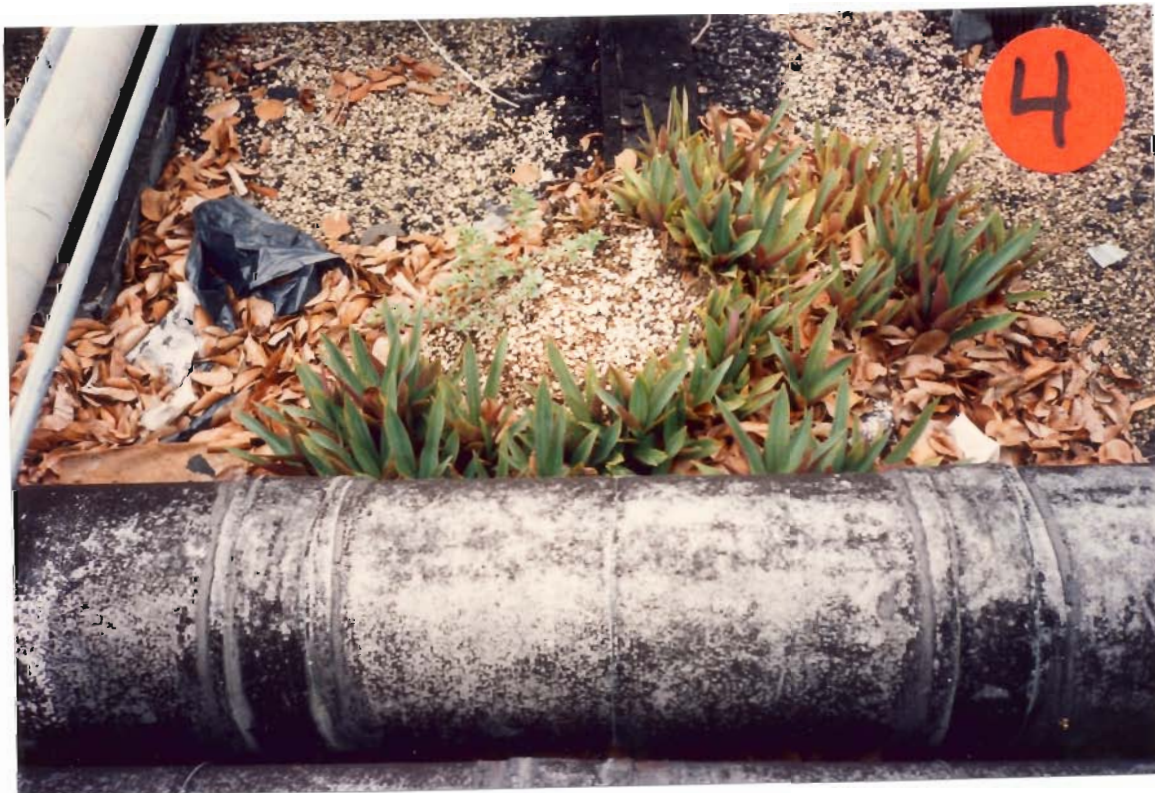
Photographs 4 & 5: Accumulated Debris And Plants On Roof Of School
