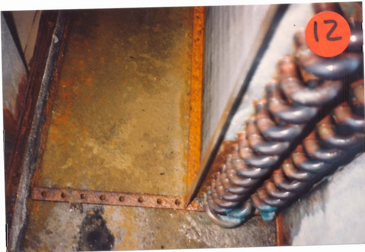
Photograph 12: Very Dirty And Rusty Condensation Pan
